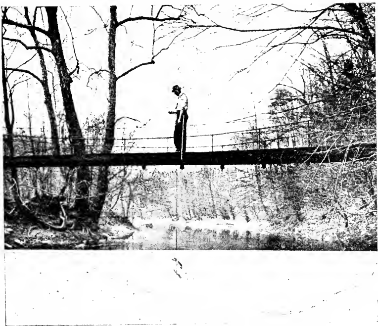
FIG. 24.—Typical Gauging Station for Bridge Measurement.
